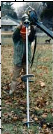
Portable equipment (hand-held or on ATV) rotates screw foundation into soil. Minimum soil disturbance results in maximum compression and uplift capacity.
